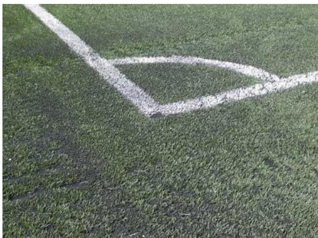
Figure 14: accumulated infill material in the corner area
