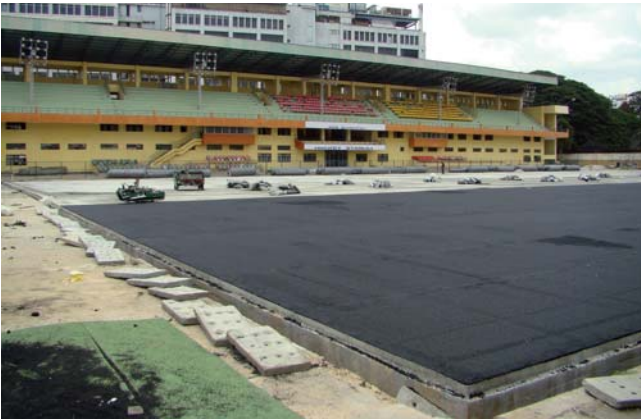
Figure 7: installation of an e-layer
