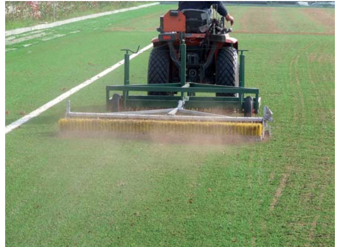
Figure 9: installation of the infill material
